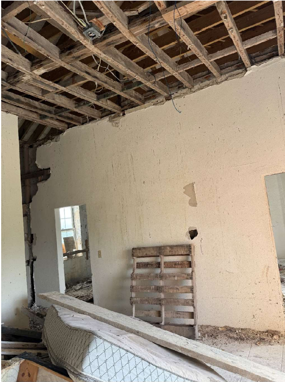
Upper-Level Existing Conditions
