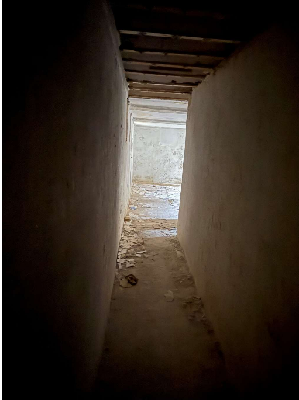
Corridor to Basement
