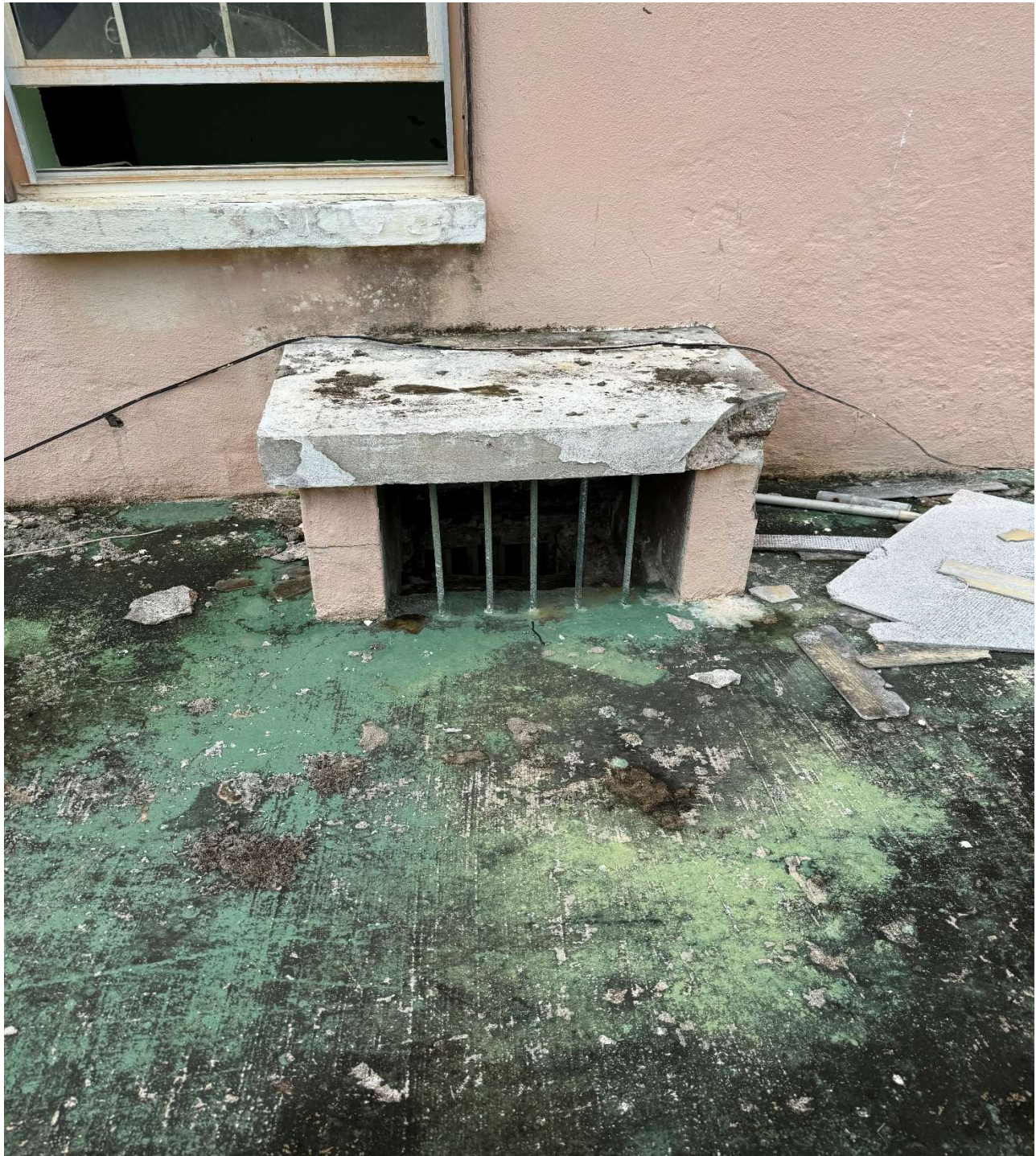
Window Well (Existing Condition)
