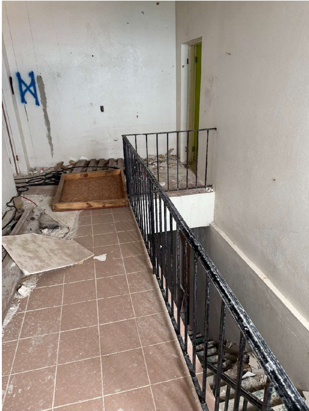
Interior Stairs (Upper Level)
