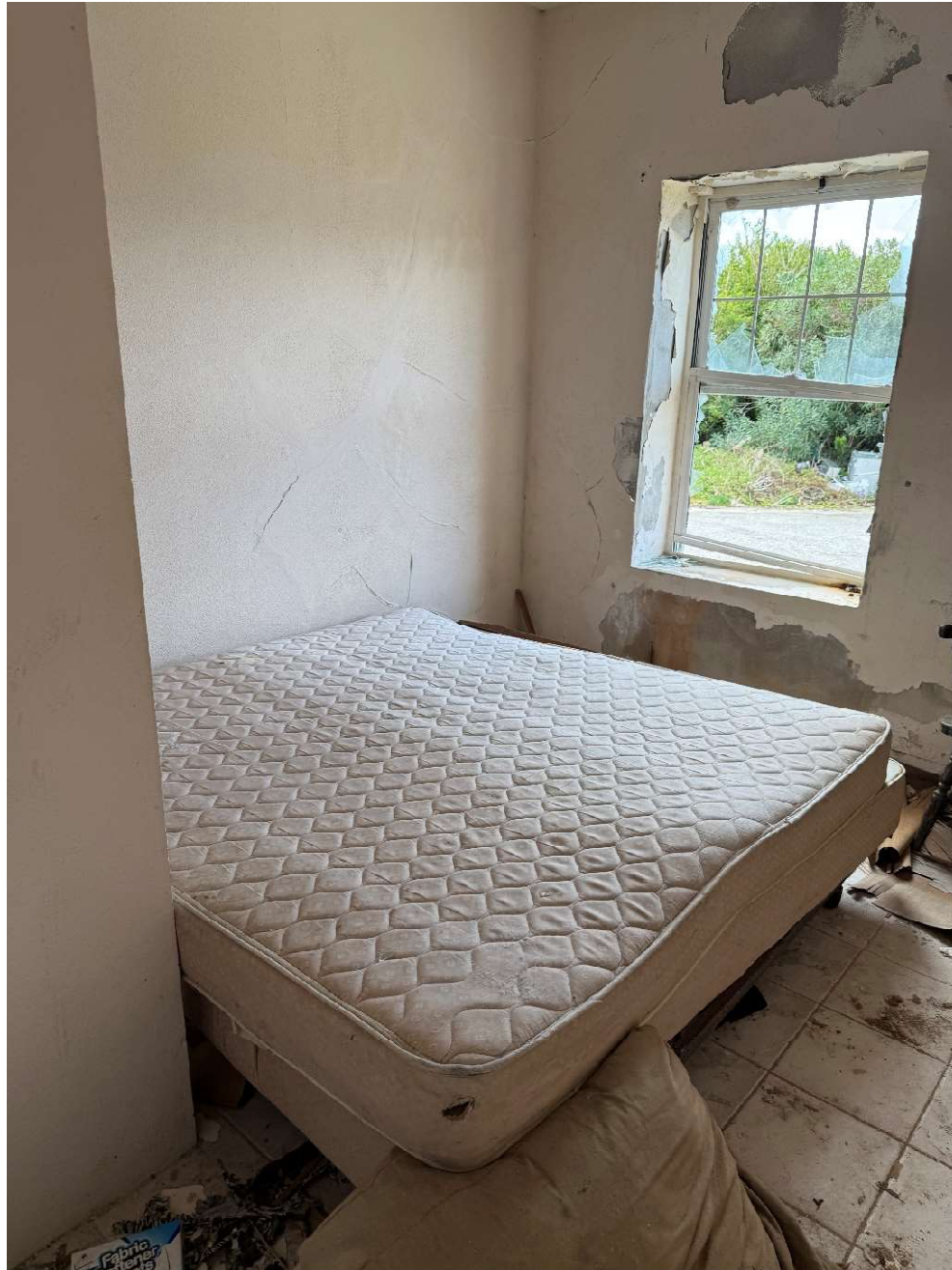
Lower West Interior Condition
