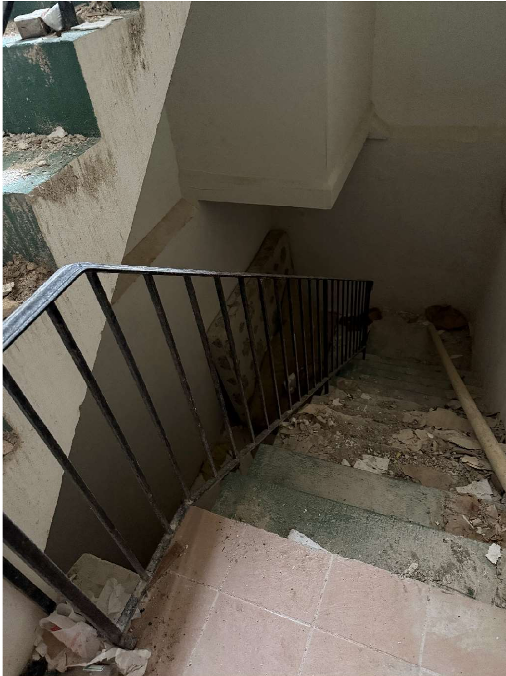
Interior Stairs Leading to Basement
