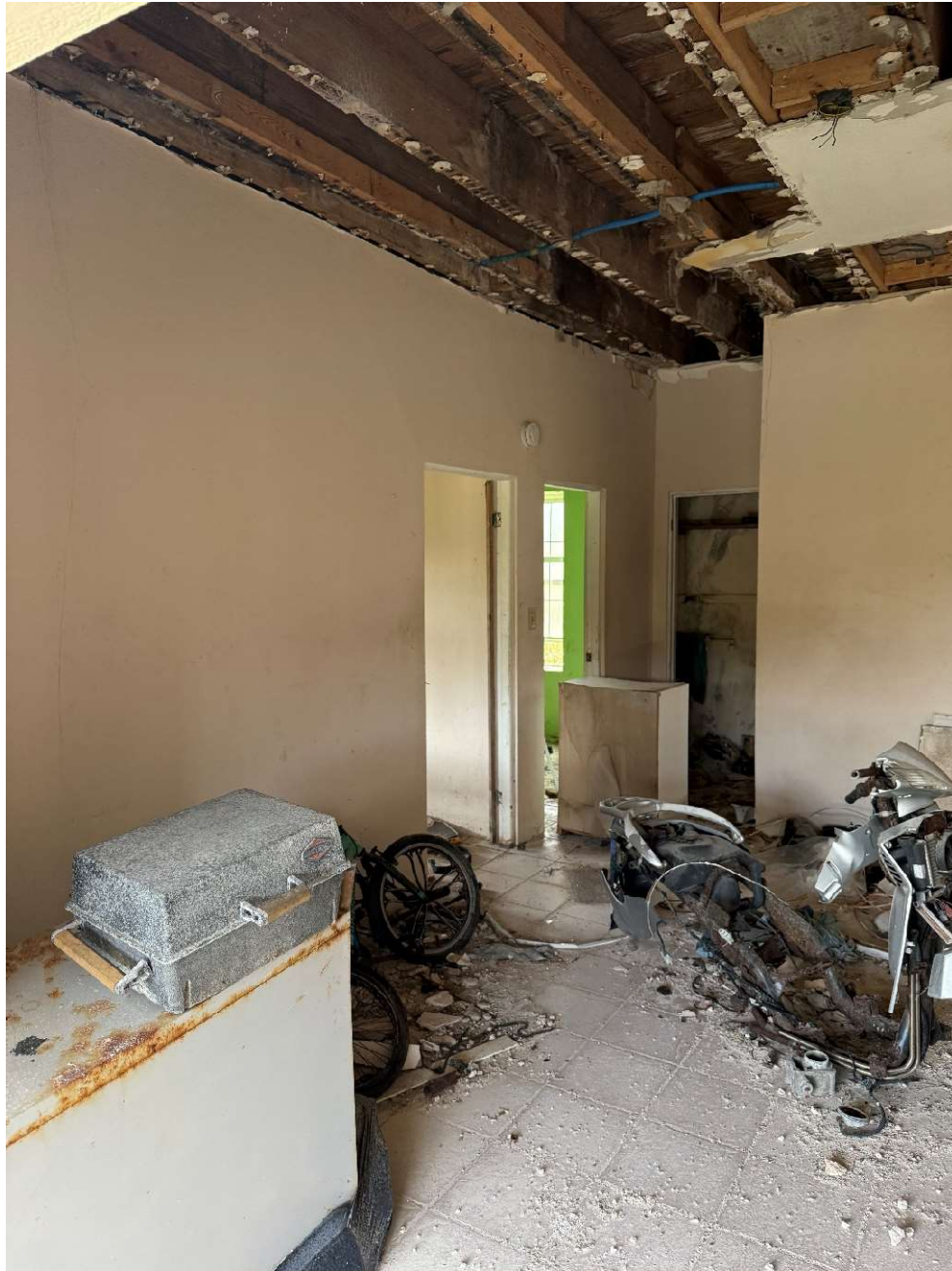
Lower West Interior Condition
